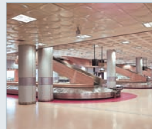
● Baggage Handling System
